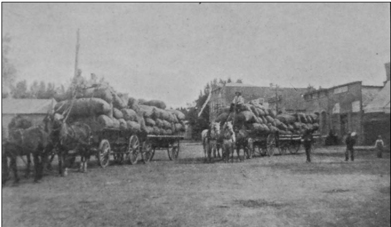
Figure 11. Wagons loaded with bags of wool stand in the middle of the 300 block of 4 th Street. The building with the awning is 301 4 th Street (5SH.1903) and the double building right of the wagon is number 307 (5SH.1904). The two-story Dunn Block (5SH.1901) is in the distance and the building at the left edge of the image may be the Saguache Crescent building. Courtesy of Saguache County and the Northern San Luis Valley , ca. 1908, in Western History and Genealogy Department, Denver Public Library, Denver, Colorado.
