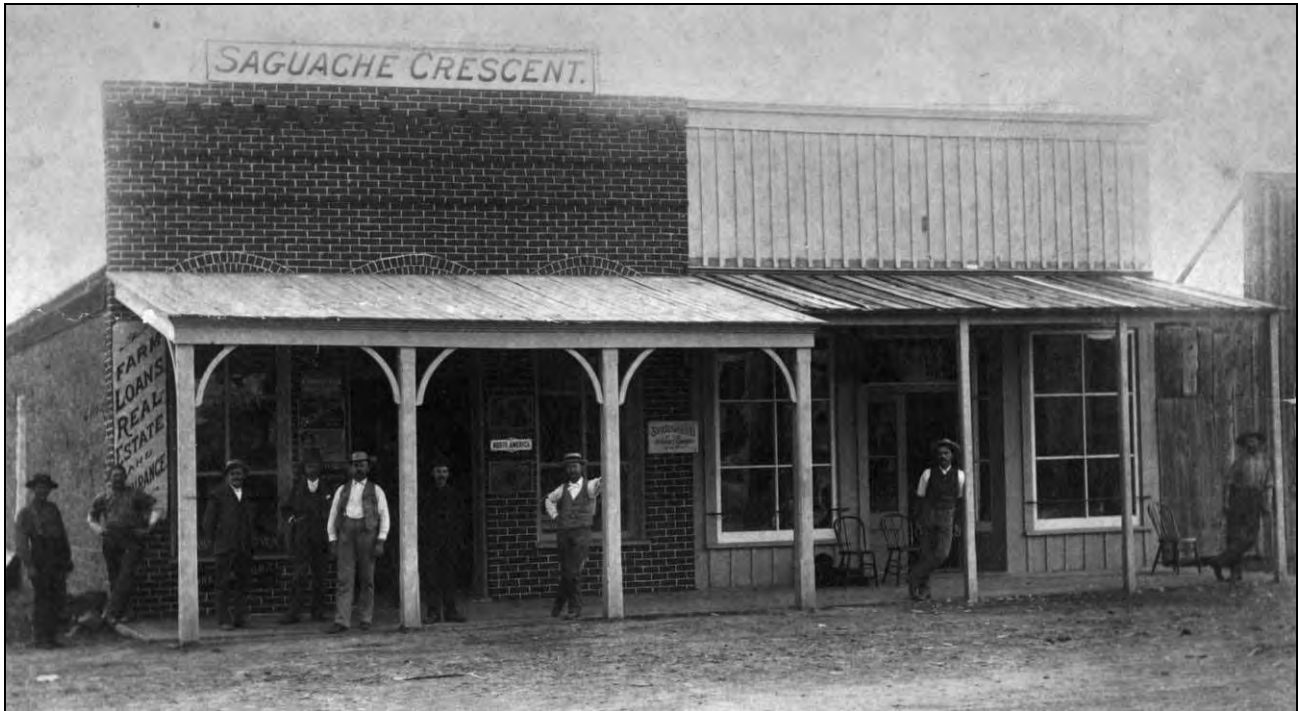
Figure 8. This ca. 1890s view east-southeast shows the Saguache Crescent building at 316 4th Street (5SH.1898). The north (left) section of the two false front sections is adobe faced with brick. Courtesy of Western History and Genealogy Department, Denver Public Library, photograph collection, L.R. Phillips, image number X-13450, ca. 1890s, Denver, Colorado.
