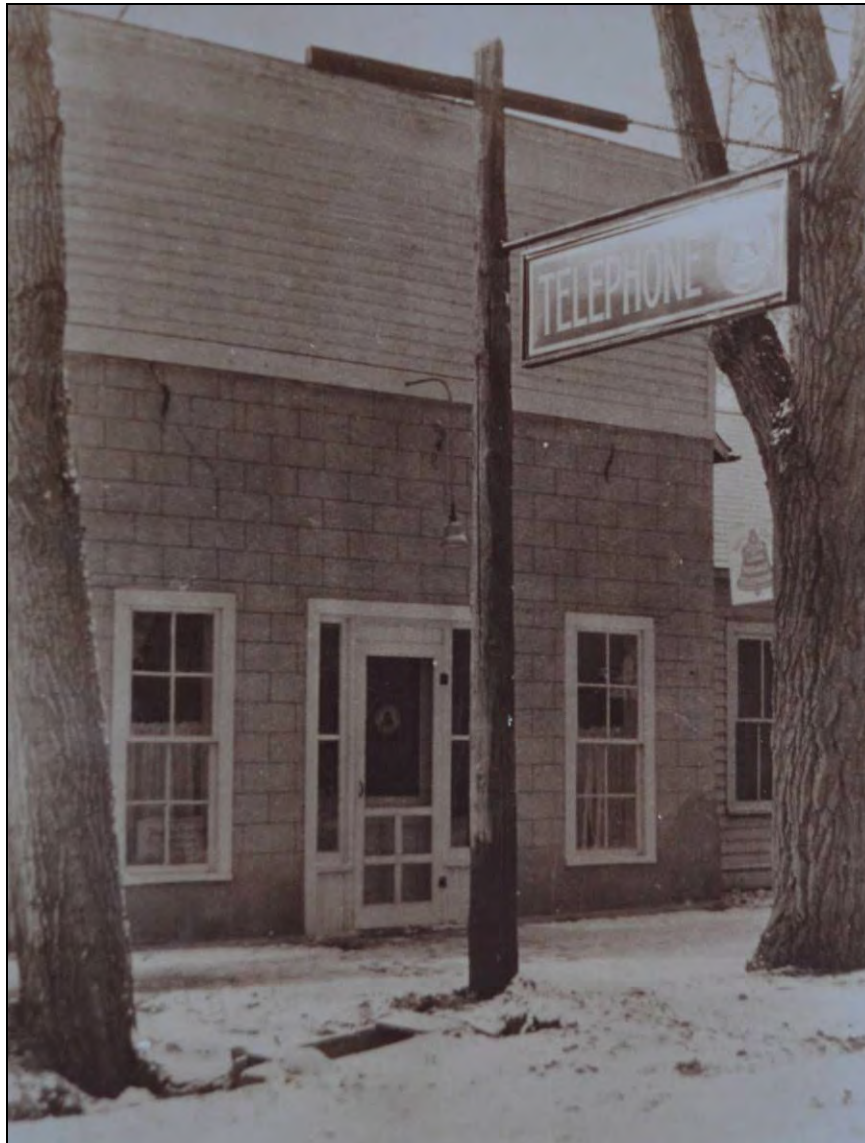
Figure 22. The town's telephone exchange, pictured here in a 1926 photograph, was housed in an adobe building with a false front at 435 San Juan Avenue (5SH.3644). Courtesy of Roger A. and Marilyn K. Fenton, 1926, Saguache, Colorado.
