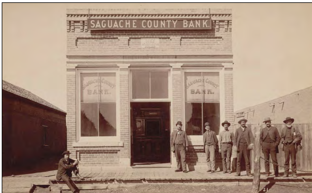
Figure 7. By 1882, the Saguache County Bank had outgrown its space in the Gotthelf and Mayer building (right) and this building at 311 4 th Street (5SH.1900) was erected to house its operations. The building plaque below the signband reads "1882 J.F. Farrington builder." The walls of 313-15 (5SH.1902) and 307 4 th Street (5SH.1904) are shown to the left and right, respectively. Courtesy Amon Carter Museum, photographic collection, image number P1976.11.226, ca. 1880s, Fort Worth, Texas.
